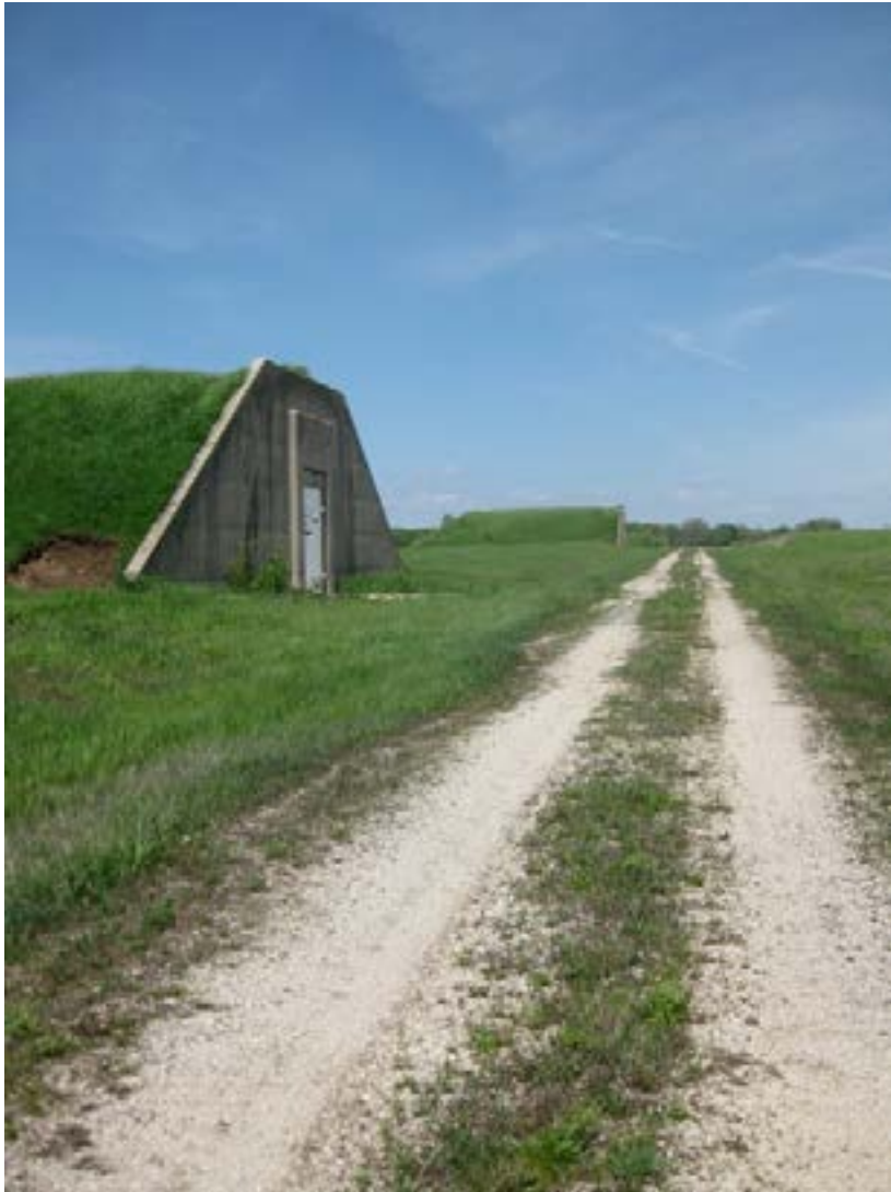
Empty storage bunkers, called igloos, on a stripped railbed at the Joliet Army Ammunitions Plant, Joliet, Illinois; photo taken by the author, David Meyerson
